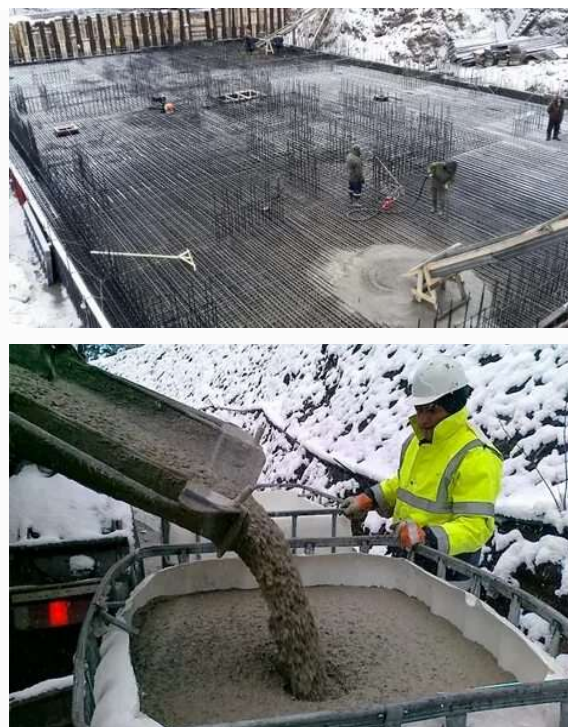
Figure 1. Winter concreting process
