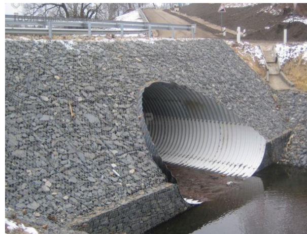
Figure 2. gabion pipes and structures for the construction of bridges and overpasses
