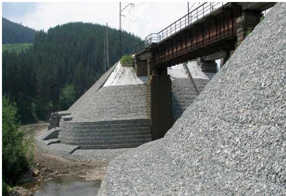
Figure 1. Geomembrane for securing the bridge cone with a gabion
